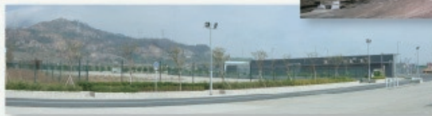
EcoPark in Tuen Mun Area 38
