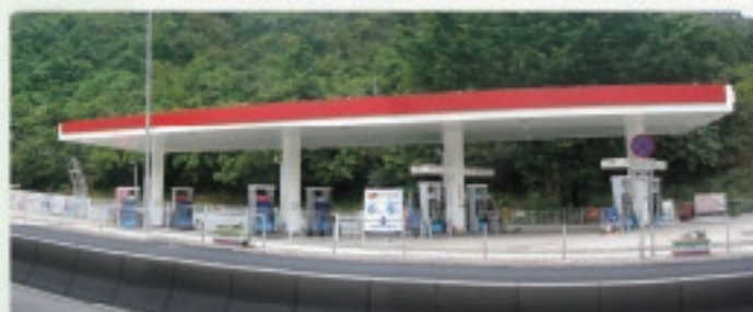
◀ A Petrol Filling Station with LPG filling facilities at Tsing Yi Road West, Tsing Yi
