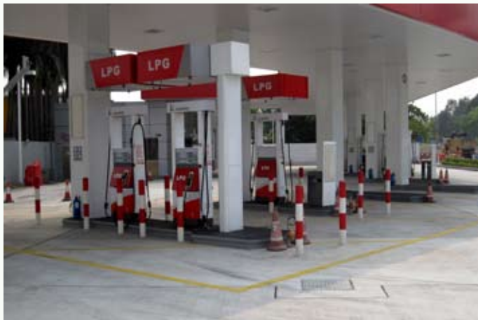
A Petrol Filling Station with LPG filling facilities at Castle Peak Road, Ping Shan, Yuen Long
