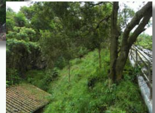
After slope works
