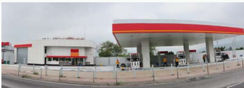
A Petrol Filling Station with LPG filling facilities at Kam Tin Road, Yuen Long
