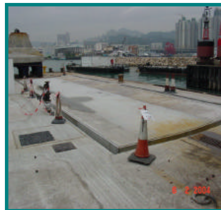
Effective Drainage System
