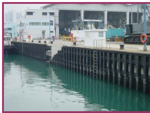
Plastic Fenders erected alongside the Seawall of GD
