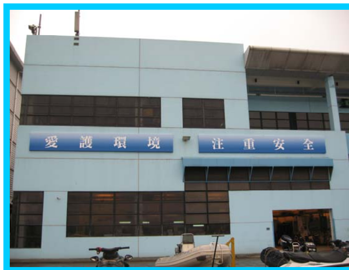
New Safety Slogan Displayed on Workshop Building
