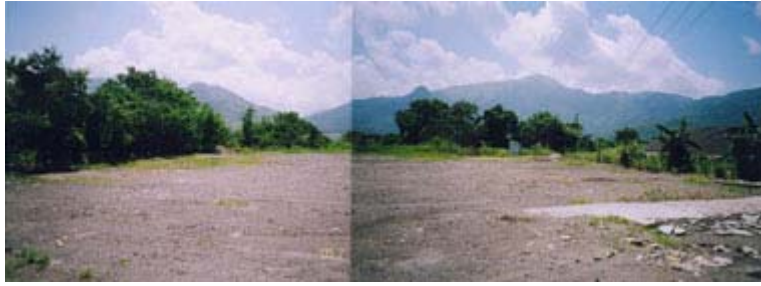
UD site cleared after taking enforcement action
