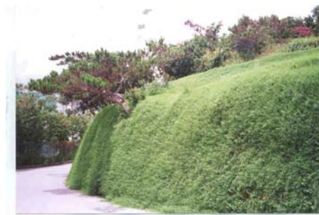
Nam Long Shan Road (after planting on shotcreted surface)
