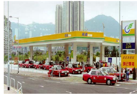
LPG filling station
