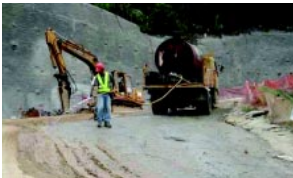
灑水以防塵土飛揚 Water spraying for dust control
