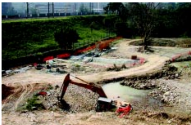
所挖出的石塊用作填料 Excavated rock used for filling
