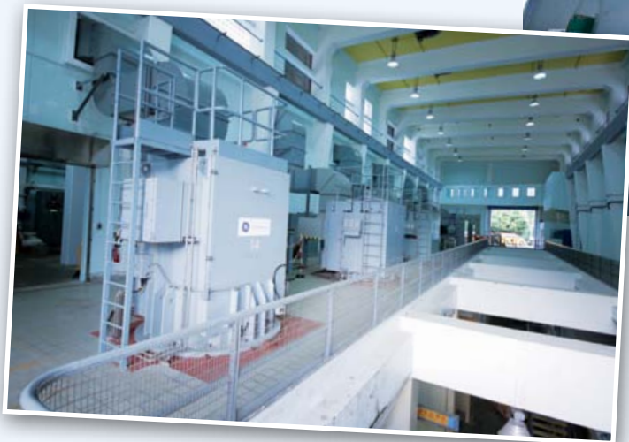
沙田濾水廠設置新泵 New pumpset in Sha Tin Water Treatment Works
