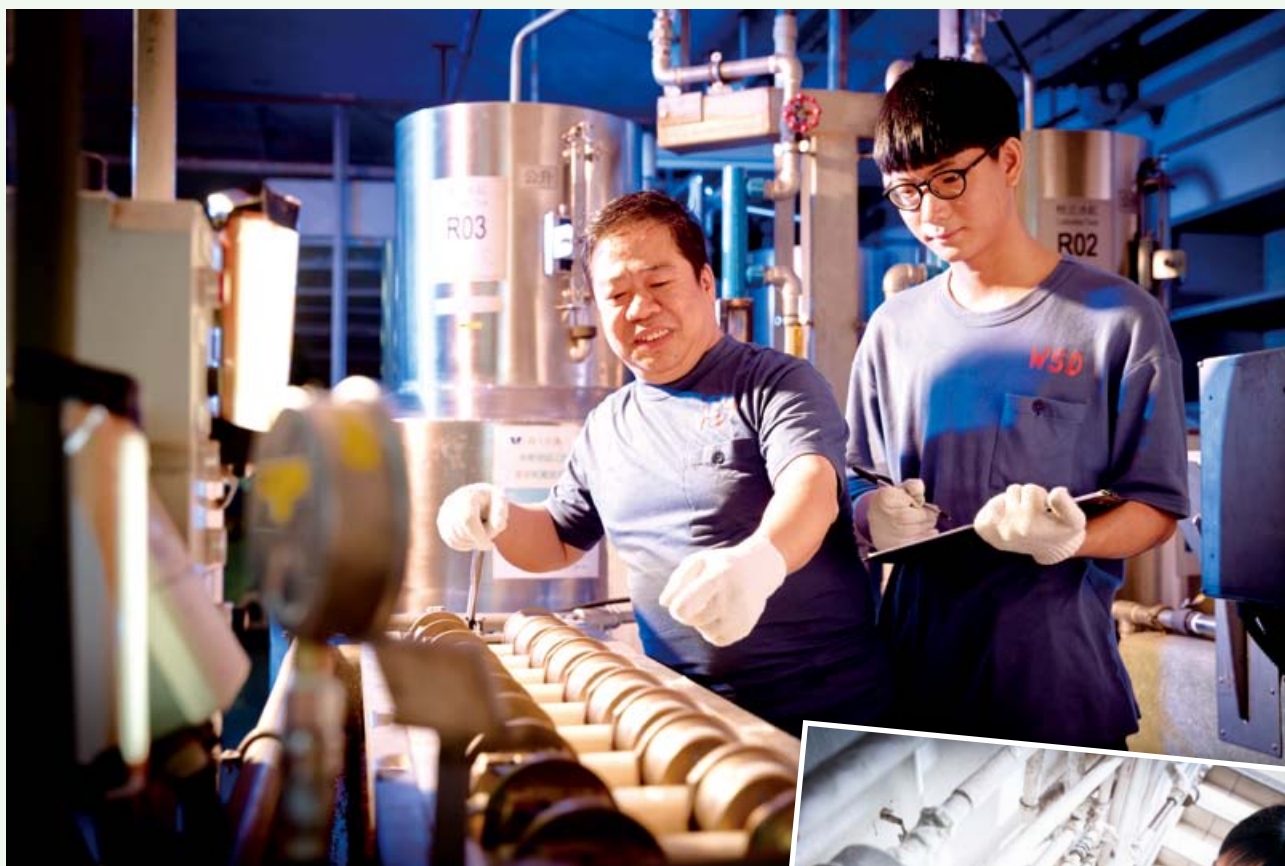
進行水錶測試 Meter testing in process
