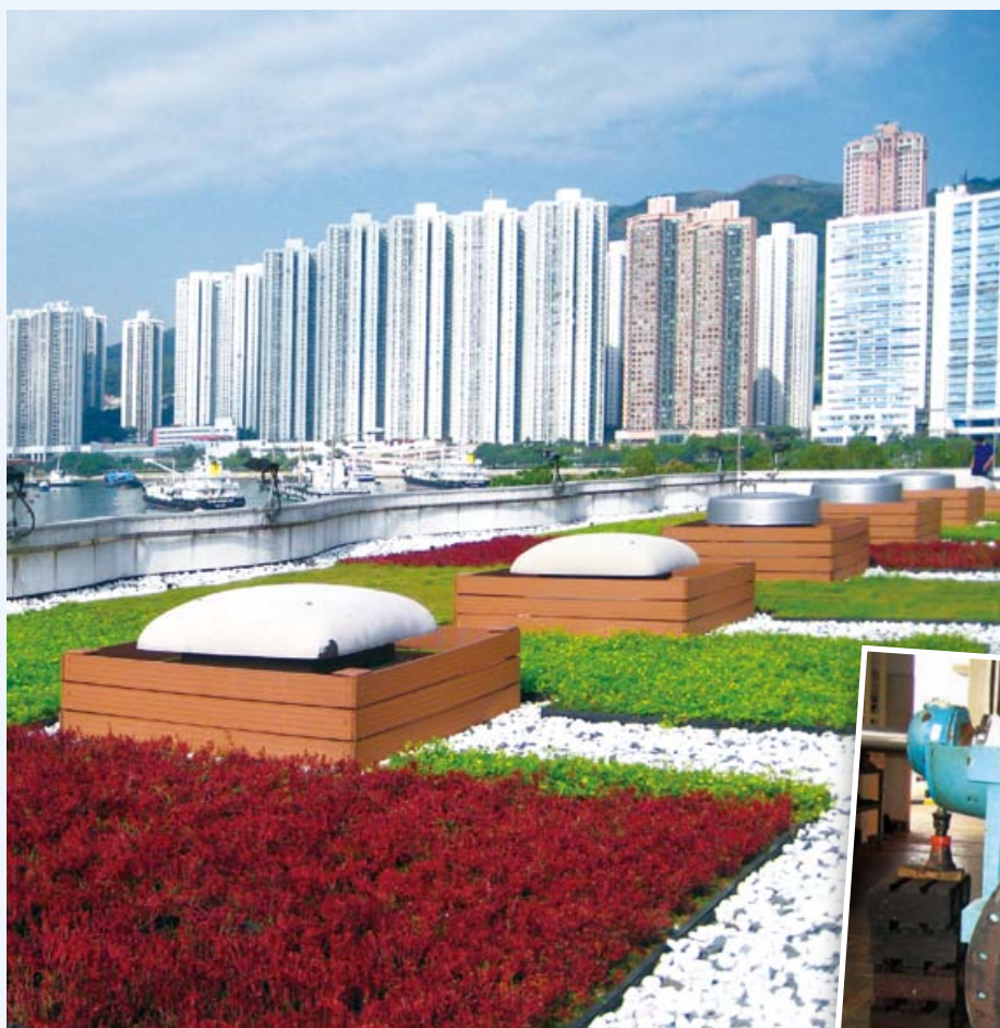
抽水站的綠化屋頂 Green roof on a pumping station
