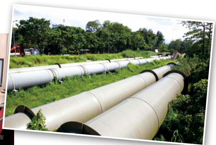
東江原水輸水管道 Pipeworks of Raw Water Supply from Dongjiang
