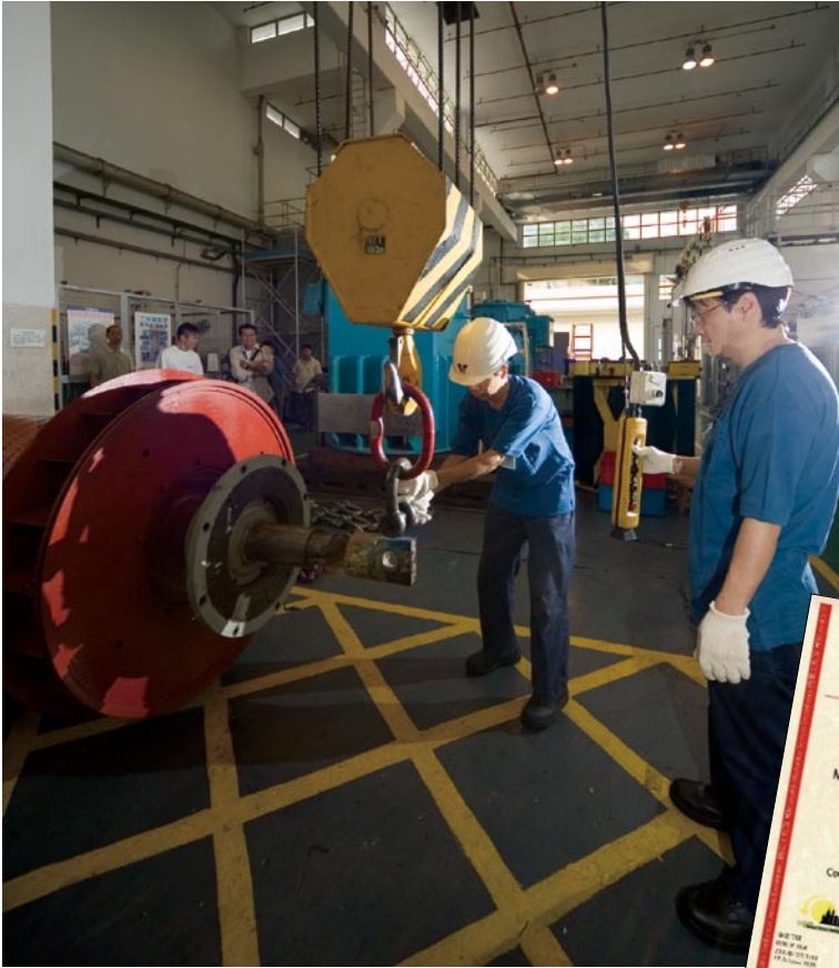
水務署龍翔道機電工場。 WSD Lung Cheung Road Mechanical and Electrical Workshop.
