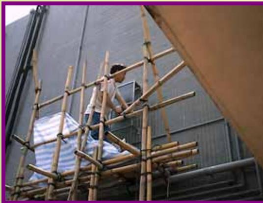
Install exhaust fans to replace air-conditioners in lift machine rooms
