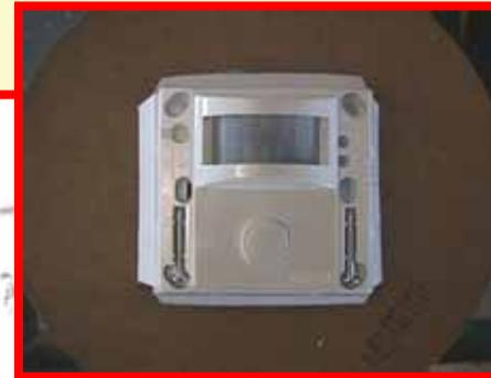
**Install infrared sensors switch to control lighting in plantrooms**
