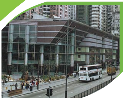
Separating the residential building and carriageway with a shopping mall to reduce the traffic noise nuisance caused to nearby residents.
