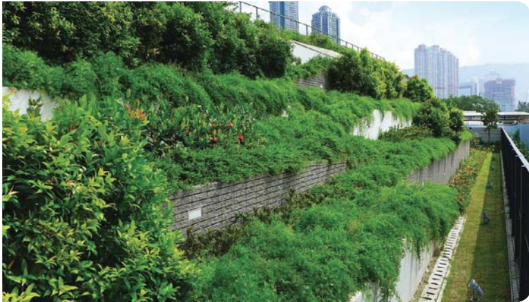
九龍城二號污水泵房的垂直綠化 Vertical greening at Kowloon City SPS No. 2
