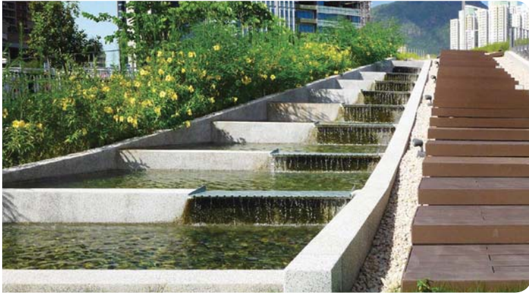
九龍城一號污水泵房的水景 Water feature at Kowloon City SPS No. 1
