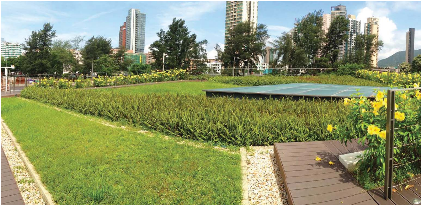
九龍城二號污水泵房的綠化天台 Green roof at Kowloon City SPS No. 2
