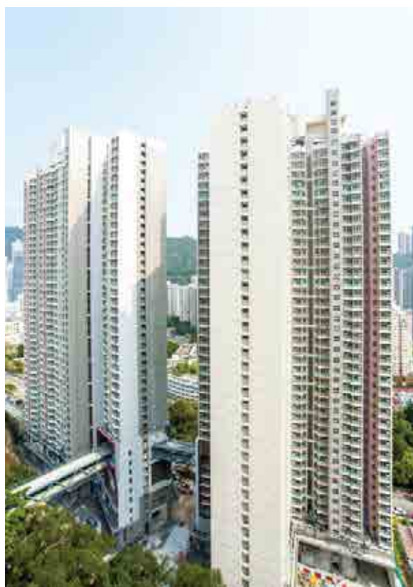
葵联邨葵逸楼和葵悦楼
