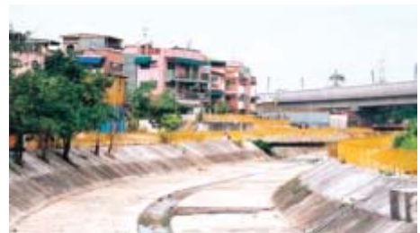
屯門河上游仍未敷設污水渠 The upper reach of Tuen Mun River is not yet sewerred
