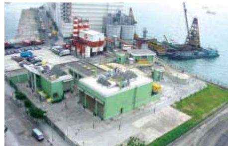
柴灣污水廠的污水已轉流至淨化海港計劃的排污隧道網絡 Sewage from Chai Wan Preliminary Treatment Works has been diverted to the tunnel network of HATS
