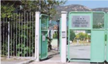
建議中會擴充梅窩污水處理廠以處理來自南大嶼山的污水 The upgrading of Mui Wo STP has been proposed to treat also the flow from the south of Lantau
