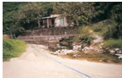
未敷設排污渠的大浪灣腹地仍是泳灘的潛在污染源 The unsewered hinterland of Big Wave Bay is still a potential pollution source for the beach
