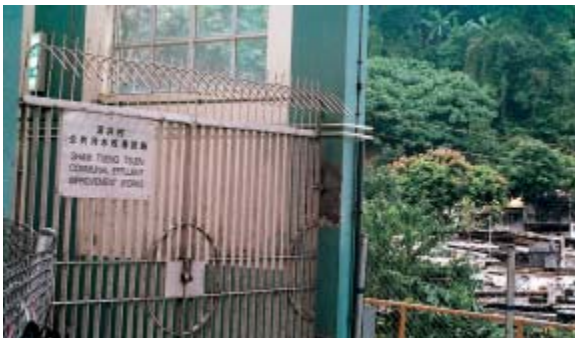
深井的臨時污水廠收集及處理部分流入深井明渠的廢水 The interim sewage treatment plant at Sham Tseng collects and treats part of the wastewater discharged to Sham Tseng Nullah
