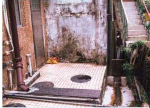
村屋化糞池滿溢時會影響附近泳灘的水質 Overflow from septic tanks would adversely affect the beach water quality
