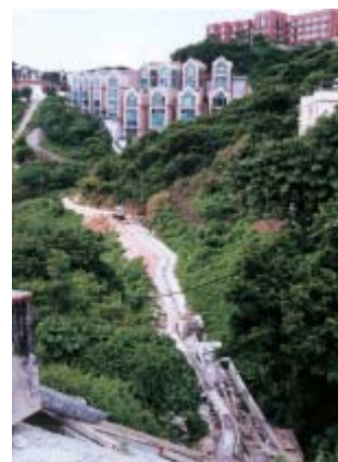
銀線灣區的渠務工程 Construction of sewerage system for the Silverstrand area
