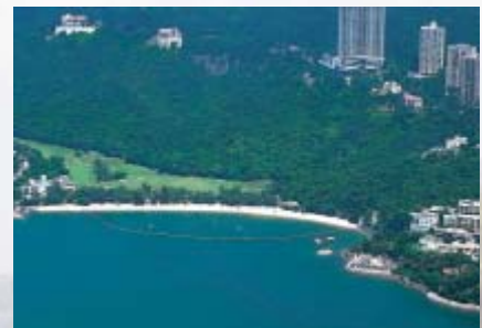
深水灣腹地現已完全接駁至排污渠 The hinterland of Deep Water Bay is now completely sewered
