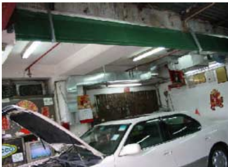
應用於小型維修車房的活性炭除味系統 Real Application in a Small Garage
