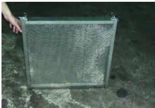
活性炭濾層 Activated Carbon Layer
