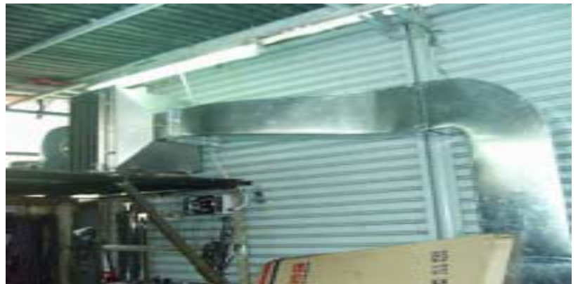
應用於中型維修車房的活性炭除味系統 Real Application in a Medium Garage
