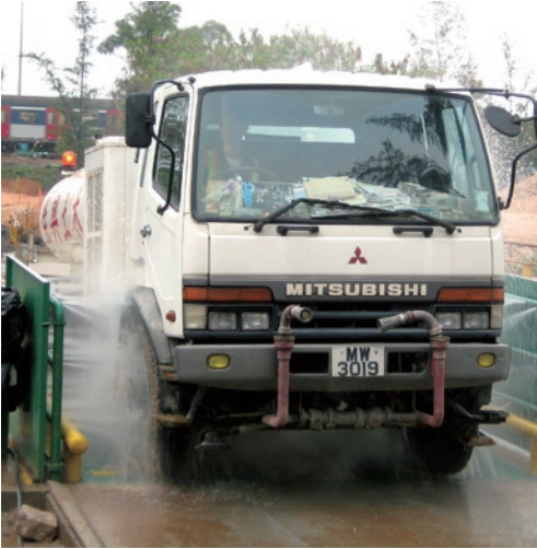
地盤出口的洗轆設施 Automated wheel-washing facility at site exits
