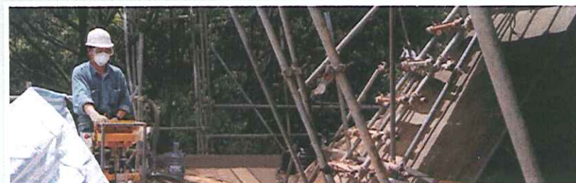
在斜坡工程中使用物料覆蓋措施 (在鑽孔時使用帆布覆蓋和灑水以減少塵埃散佈) Typical dust-control measures covered in slope engineering works (use tarpaulin sheets and water spraying to suppress dust generated from drilling)
