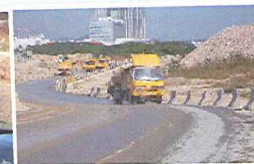
經常於工地範圍灑水以控制泥塵散佈 Regular water spraying on sites for dust control
