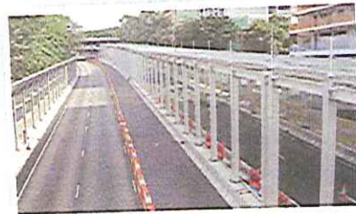
0 4 2 3 4 5 6 7 8 9 Noise barriers and semi-noise enclosures
