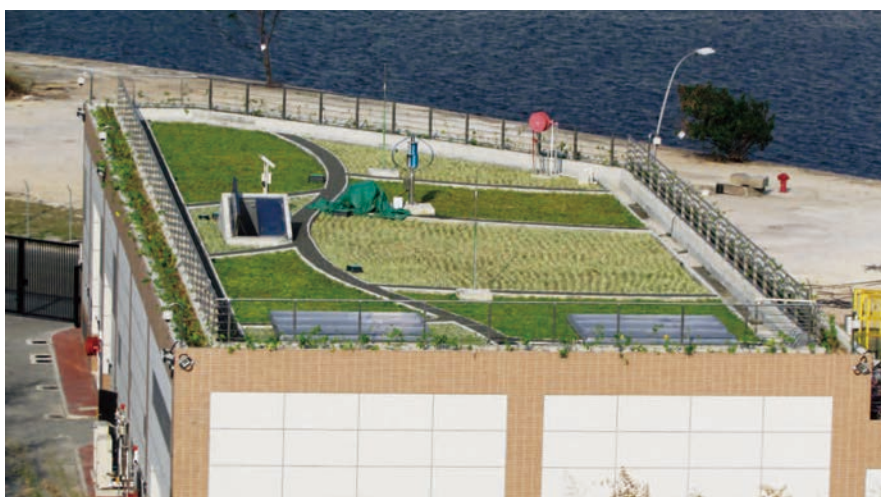
啟德發展計劃 — 前跑道南發展項目的前期基礎設施第一期工程 Kai Tak Development — Advance Infrastructure Works for Developments at the Southern Part of the Former Runways, Stage 1 污水泵房的屋頂綠化 Green roof of sewage pumping station
