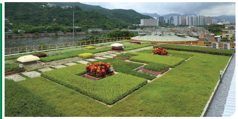
● 沙田污水處理廠的綠化天臺 Green roof at Shatin Sewage Treatment Works
