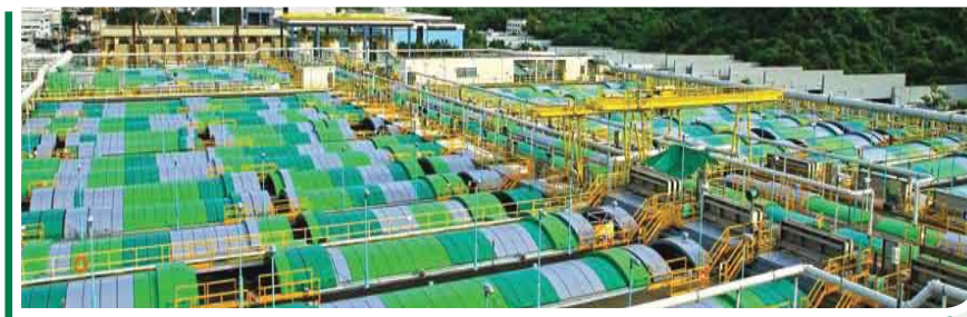
已覆蓋的沉澱池 Covered sedimentation tanks
