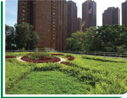
● 兆康污水泵房的綠化天台 Green roof at Siu Hong Sewage Pumping Station
