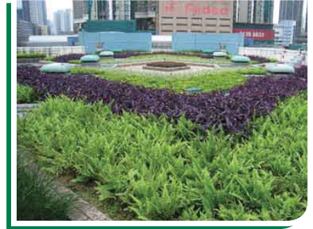
● 水船街污水泵房的綠化天台 Green roof at Water Boat Dock Sewage Pumping Station
