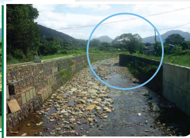
● 修改河道岸線以保育原有樹木 Re-alignment of river for preserving existing trees
