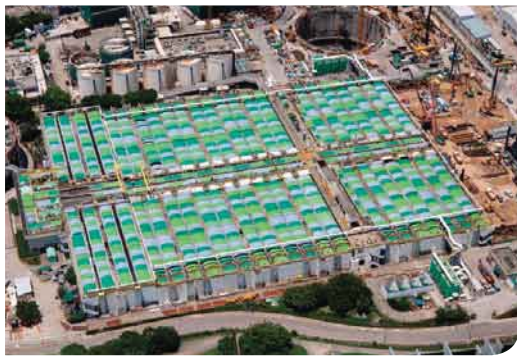
◆ 密封式沉澱池 Covered Sedimentation Tanks
