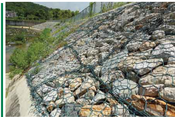
● 在河道內兩旁鋪設石籠 Rockfill mattresses at embankments of the trained river channel
