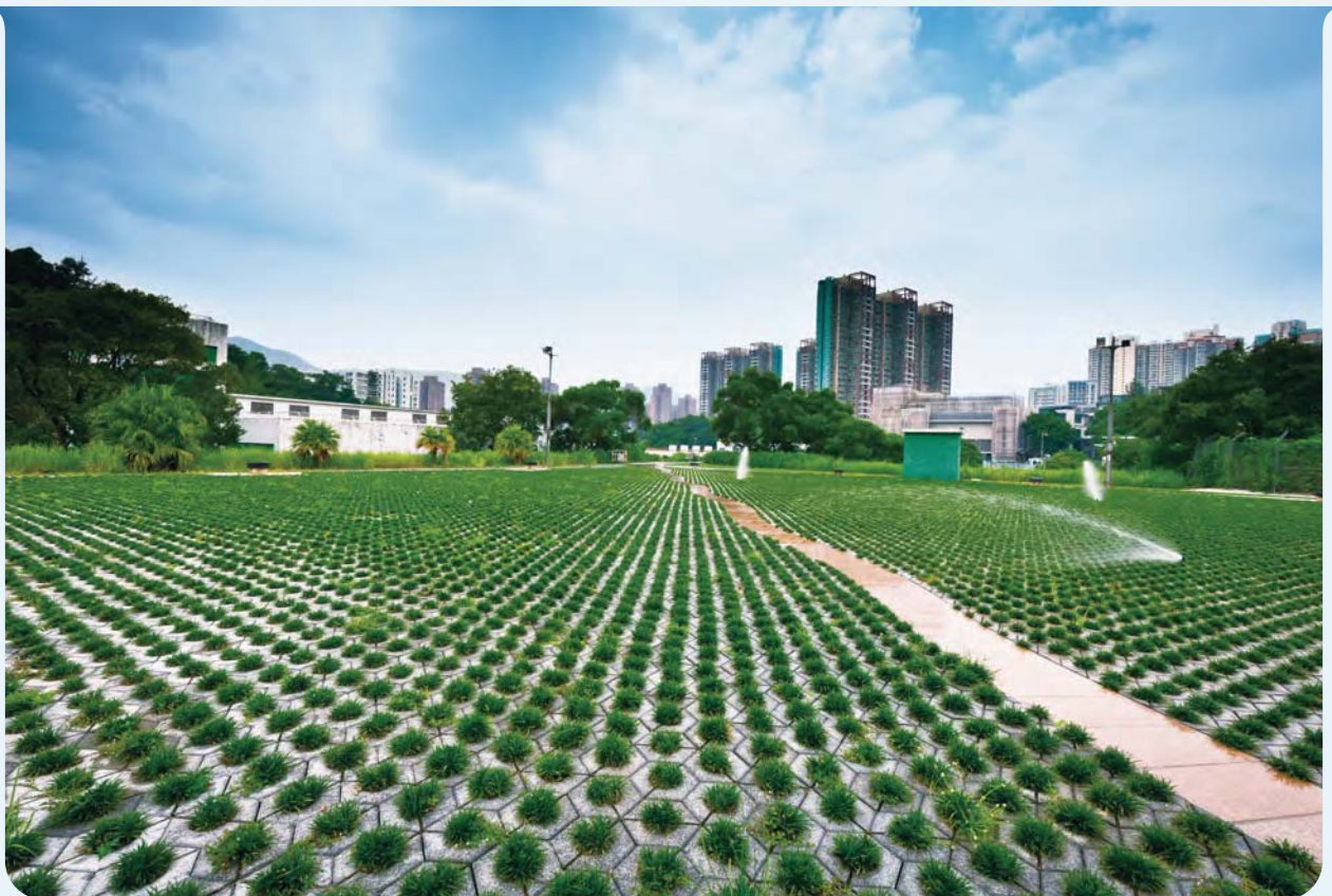
屯門濾水廠內清水池的綠化屋頂。 The green roof of the clear water tank in Tuen Mun Water Treatment Works.
