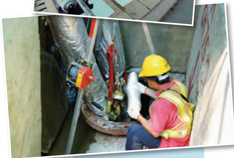
大口徑水管修復工程 Pipe rehabilitation work of large diameter pipe
