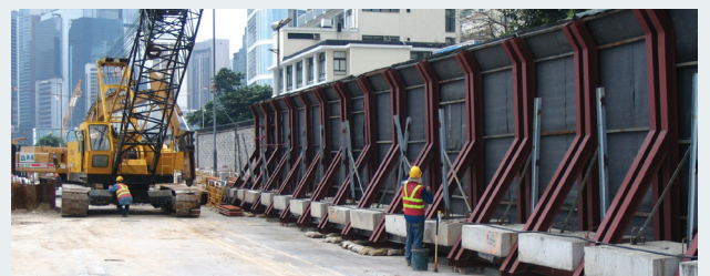
臨時隔音屏障 Temporary noise barriers
