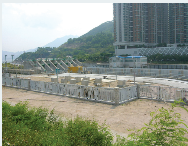
將軍澳的淤泥清理裝置 Desilting Compound at Tseung Kwan O
