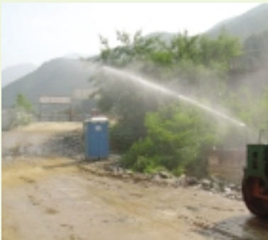
地盤運料路的灑水系統 Water spraying system at site haul road
