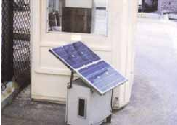
在壁屋監獄更亭安裝的太陽能電風扇系統 A solar energy electric fan system installed at a guard kiosk in Pik Uk Prison
