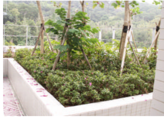
Greenery garden on the roof-tops of Kowloon Command Headquarters and Kowloon Tong Fire Station-cum-Ambulance Depot (left) and Braemar Hill Fire Station (right)
