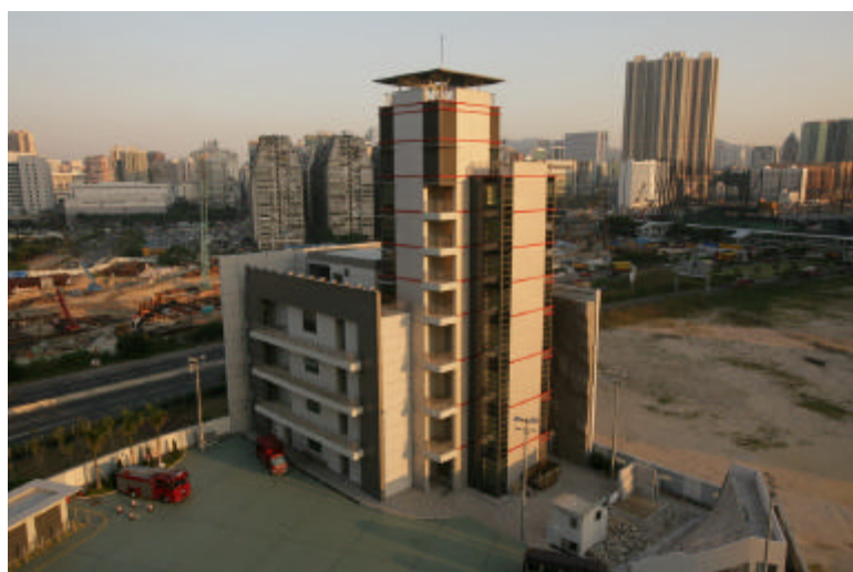
西九龍救援訓練中心 The West Kowloon Rescue Training Centre
