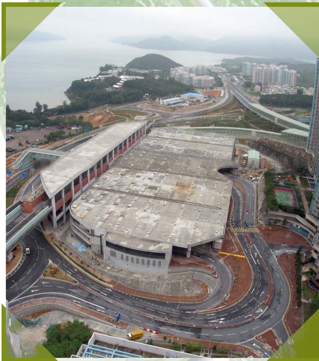
為烏溪沙站發展項目設置隔音屏障 Noise Barriers for Wu Kai Sha Station Development
