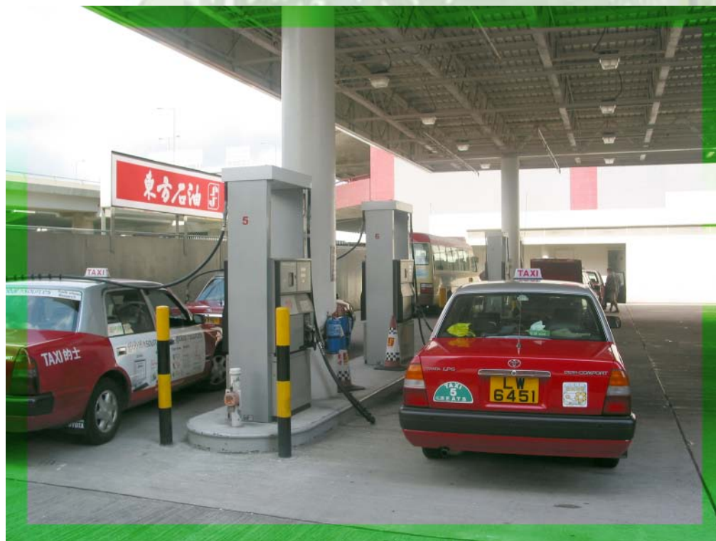
在渣華道興建具備石油氣加氣設施的加油站 A Petrol Filling Station with LPG filling facilities at Java Road
